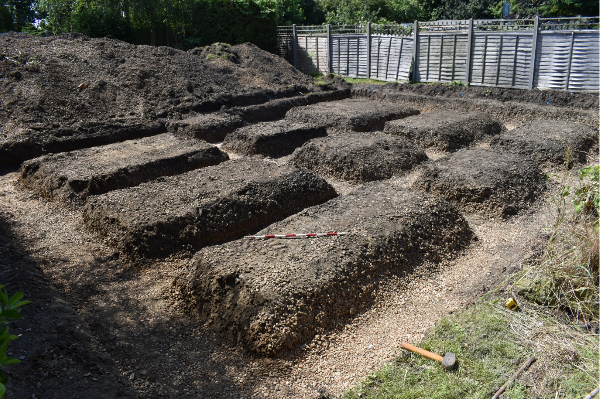
Plate 6. Foundation trenches completed (looking SW)
