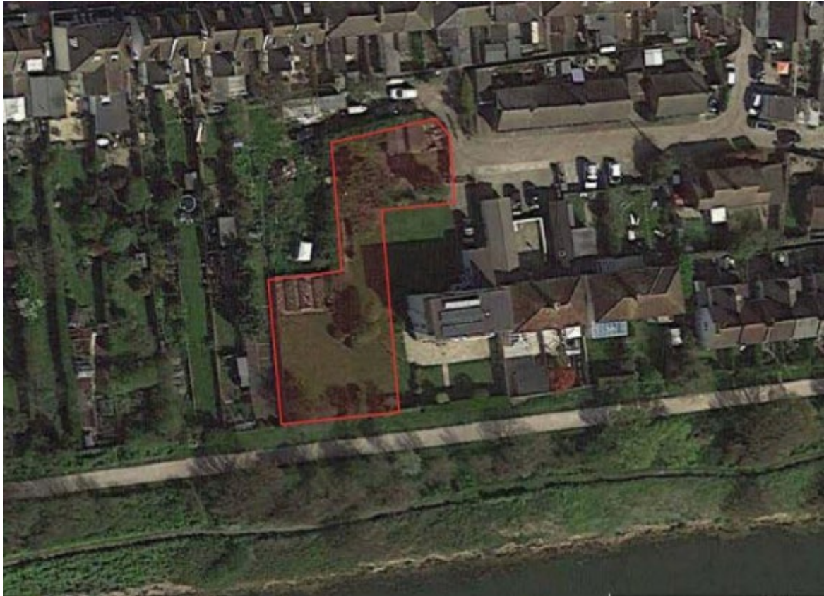
AP 1. View of site 2019 (Google Earth)
